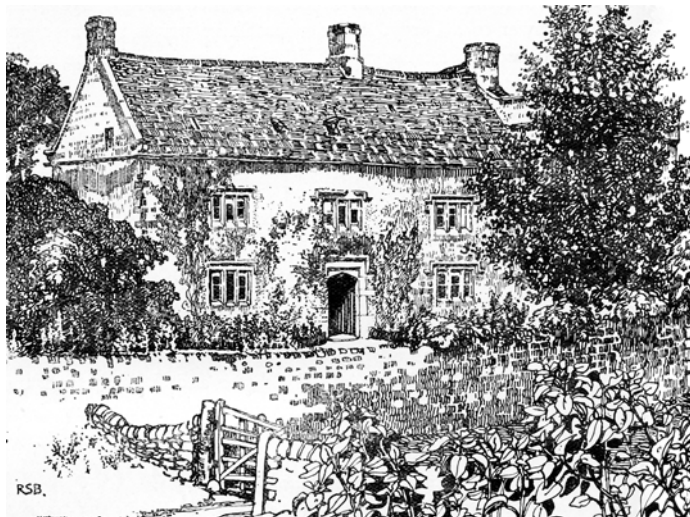
Kirkheaton Manor House (from Hodgson, 1897, reduced).
